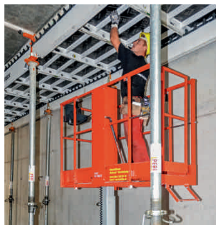
After lowering the dropheads, the central panel is removed first followed by the neighbouring panels.
