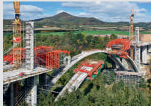
Bridge Formwork
