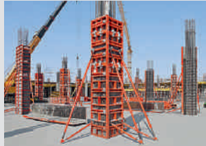
Column Formwork
