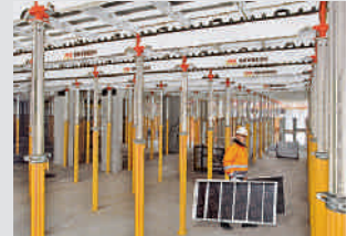
Slab Formwork
