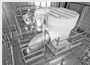
Working scaffolds industry
