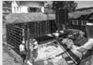
Wall formwork
