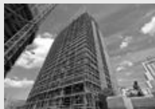
Working scaffolds facade
