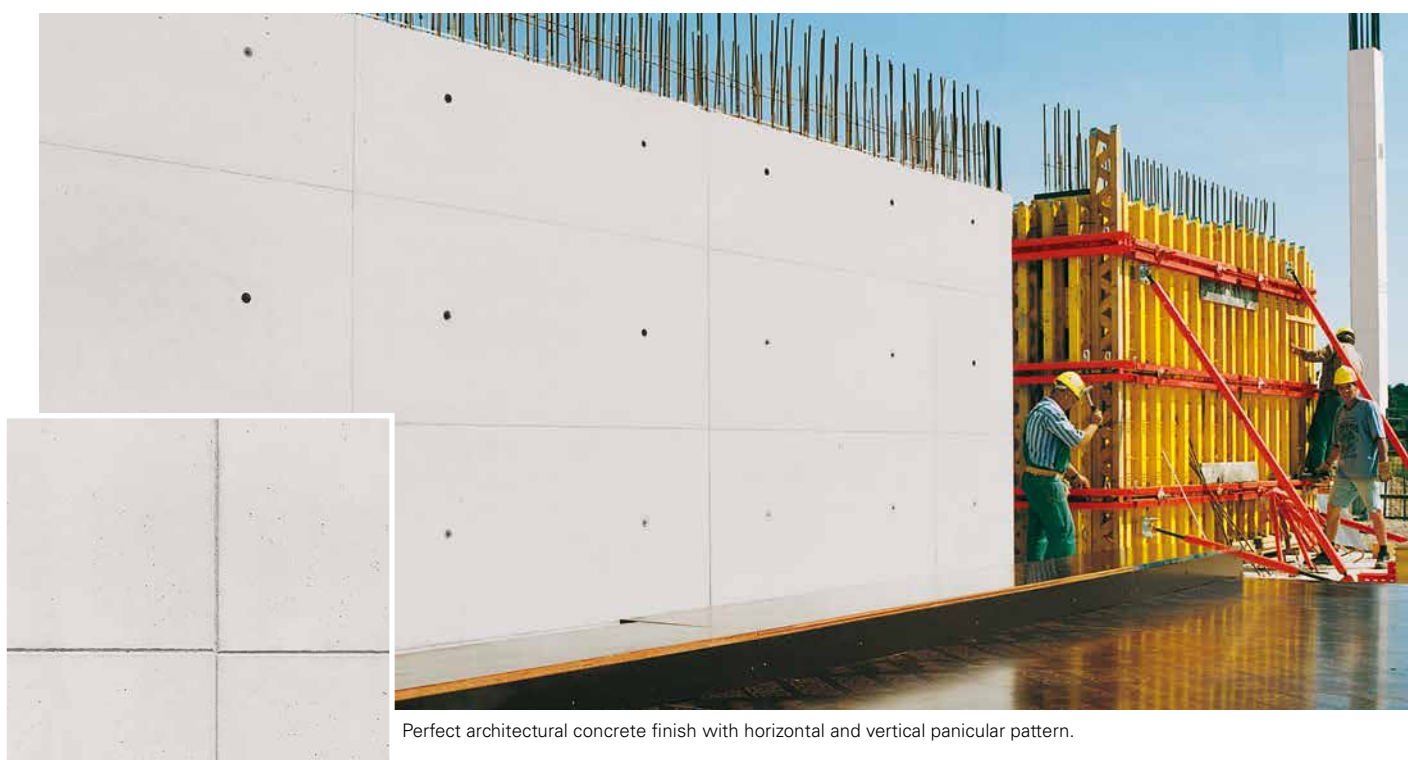
Consecration Hall, Neubiberg, Germany. VARIO with an orderly tie pattern. Formlining screwed on from the rear.
