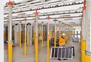
Slab Formwork
