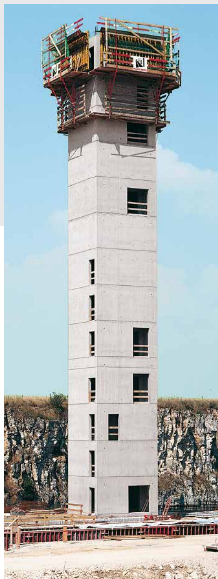
43.50 m high tower with architectural concrete with a board finish for an industrial plant.
