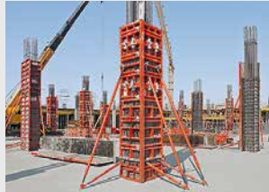
Column Formwork
