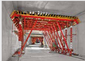
Tunnel Formwork
