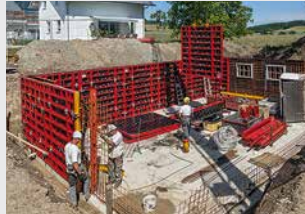
Wall Formwork
