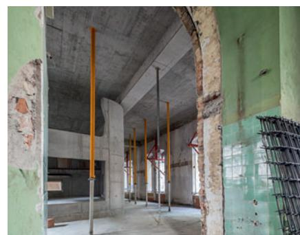
Particularly during refurbishment projects or modification work, MULTIPROP Slab Props allow working without a crane. They are easily transported and positioned by hand.
