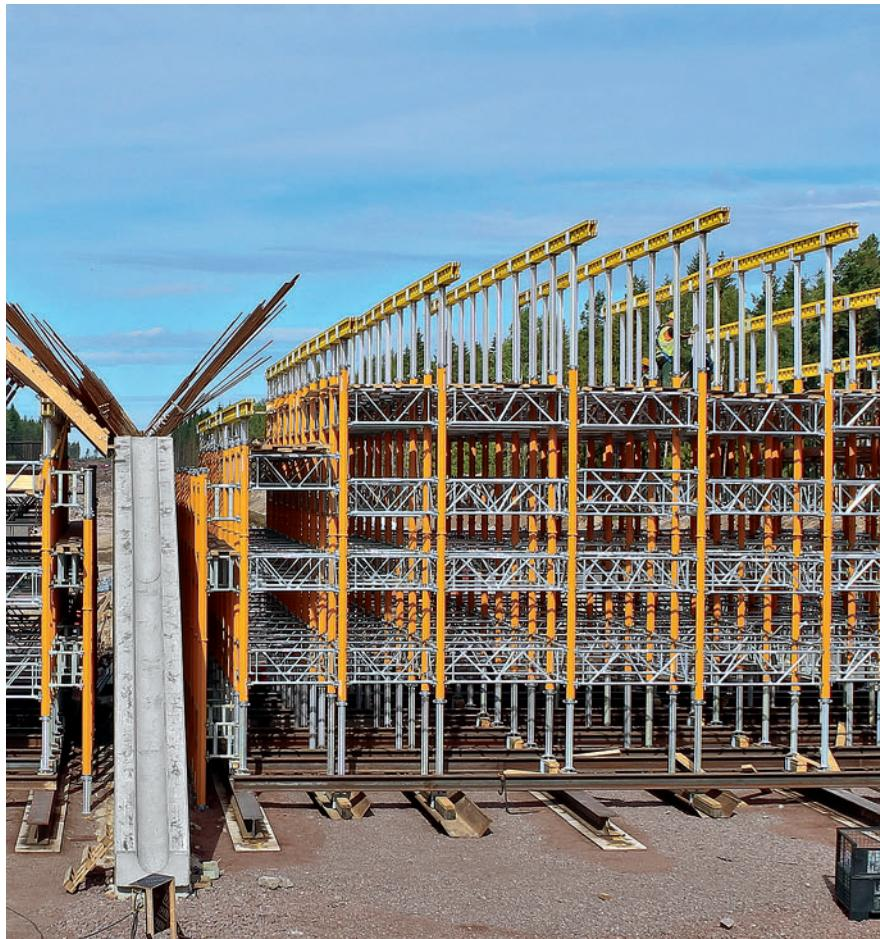
**MULTIPROP** is lightweight and, at the same time, has a very high load-bearing capacity. The props carry leg loads up to 90 kN (according to approval).
