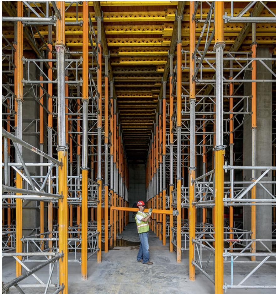
Reducing the number of props is an essential step in order to minimize the cost values for the forming of slabs. MULTIPROP Props make a significant contribution with their high load-bearing capacities.
