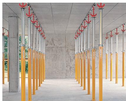
When used with SKYDECK Slab Formwork – shown here after a successful early striking – only 1 MULTIPROP Prop per 3.45 m<sup>2</sup> of slab area is required for a slab thickness up to 43 cm.
