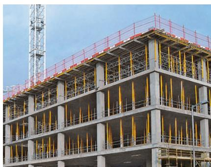
As an individual prop and braced with MULTIPROP MRK frames, the MULTIPROP Prop carries up to 90 kN per leg. Thus, MULTIPROP is also ideal for the re-shoring of slabs.
