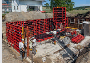
Wall Formwork
