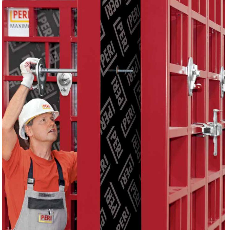
**The conical tie rod requires no spacer tubes and cones. This allows tie operations on the side of the closing formwork.**
