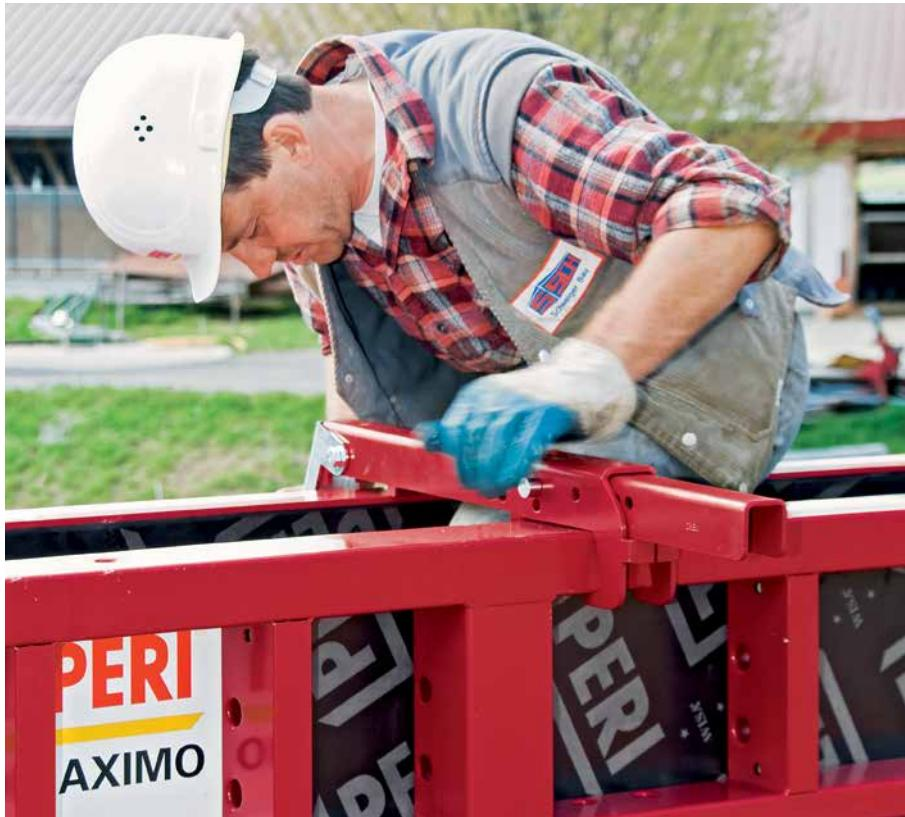
**The middle tie point brings decisive advantages when forming foundations, parapets and beams.**
