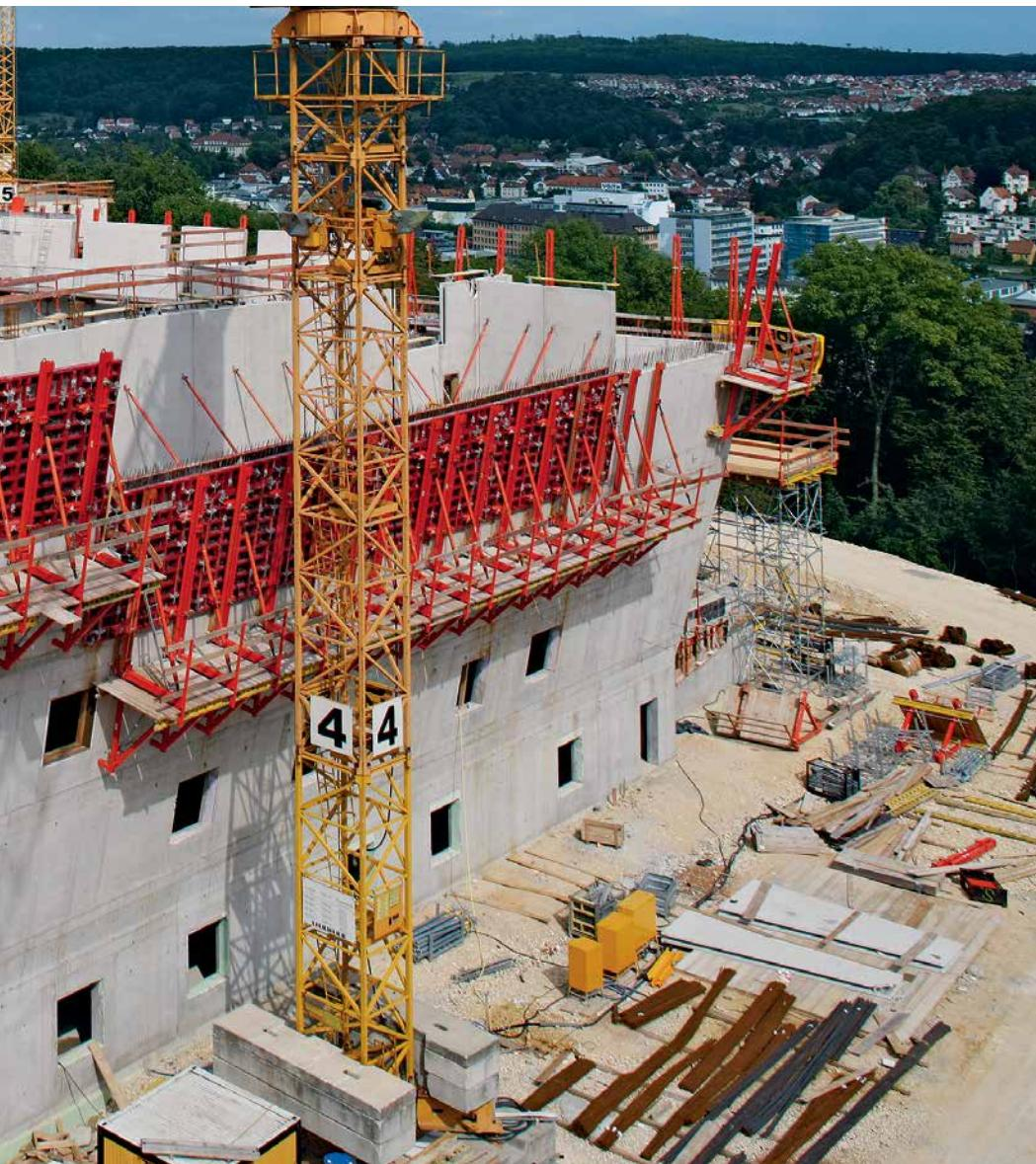
In addition to the requirement of being able to be used flexibly as well as efficiently on the construction site for all those components to be constructed, MAXIMO also fulfils the requirement to create the remaining visible concrete surfaces in high quality through the skilful selection and arrangement of the panels.
