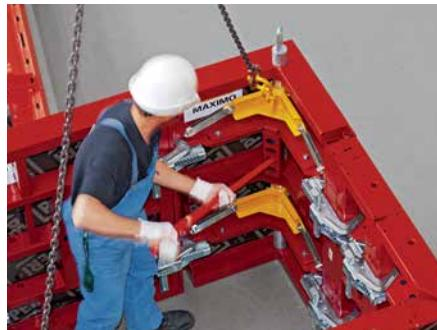
Lifting the striking mechanism with a crowbar in order to release the formwork from the concrete. It is subsequently attached to the crane.
