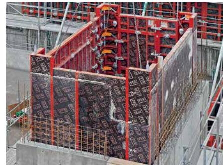
Lifting with the crane results in a 35 mm striking clearance on each side.
