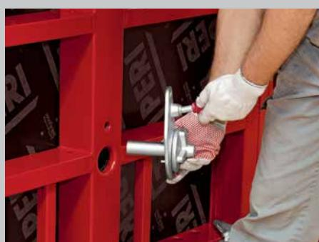
Position the Wingnut MX at the primary formwork panel and tighten the eye bolt.
