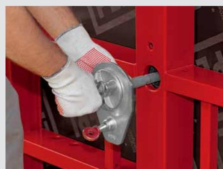
Push the MX Tie through the closing formwork into the wingnut of the primary formwork and screw in.
