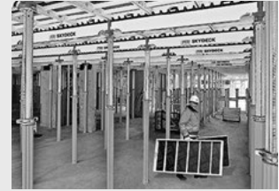
Slab formwork
