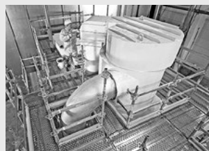
Working scaffolds industry
