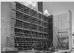
Working scaffolds construction
