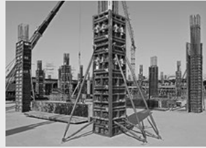
Column formwork
