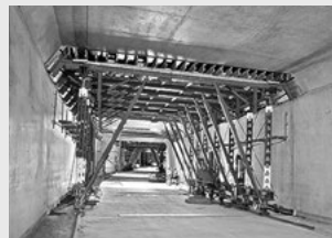
Tunnel formwork
