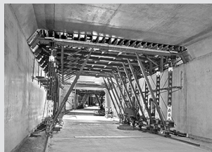
Tunnel formwork
