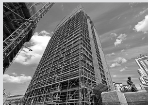
Working scaffolds facade
