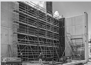
Working scaffolds construction
