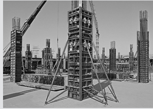
Column formwork
