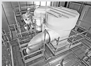
Working scaffolds industry
