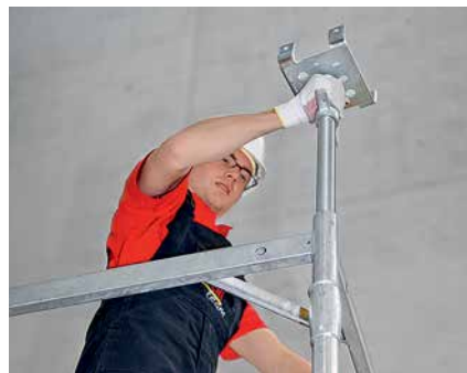
Adjust the head spindles to the required size and insert.
