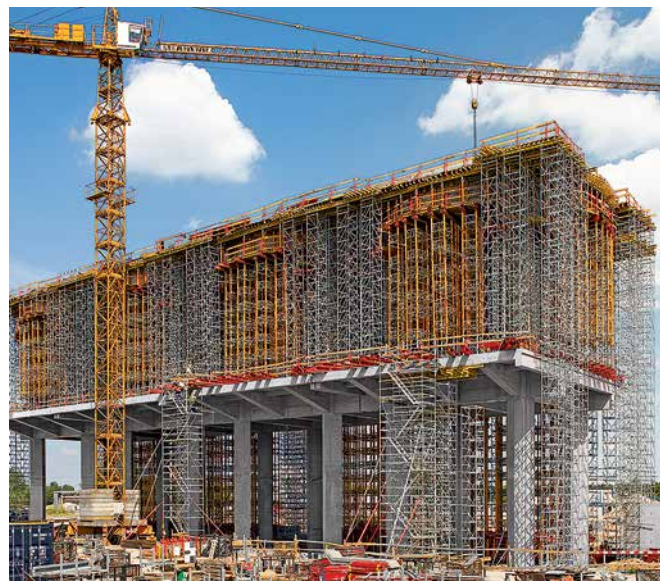
The modular MULTIPROP system and ST 100 Stacking Towers, ideally combined. Rentable SRZ and SRU Steel Walers from the VARIO wall formwork product range were used for load distribution.
