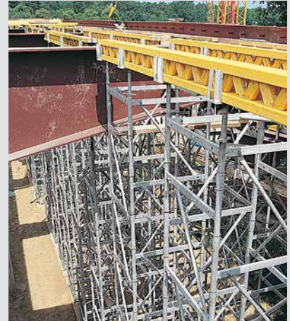
The ST 100 Crosshead Spindle securely holds one or two GT 24 Girders so they cannot tilt.
