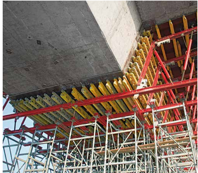
PERI framed formwork units were fixed to the bridge superstructure. In so doing, the shoring construction could then be sectionally dismantled for the next cycle.
