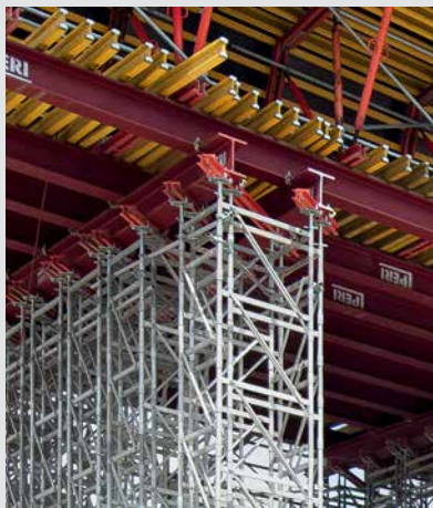
With large loads, the Head Spindle can accommodate standard PERI steel profiles, e.g. SRU or RCS profiles, as well as steel walers and other steel profiles.
