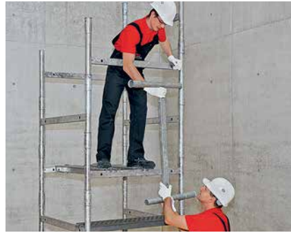
Install required number of stacking frames.
